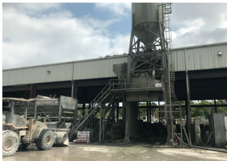
Fig 1: Original 20-year-old batch plant with high profile stacked mixer/silo.
