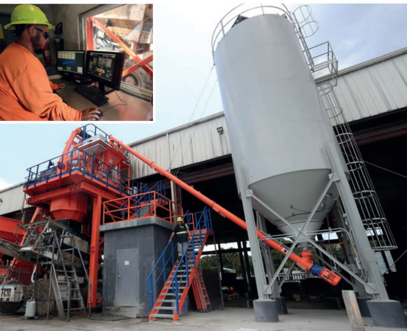
Fig 11: 700 BBL split silo contains Portland cement and fly ash. The Tucker operators are responsible for running the concrete batch plant in addition to refilling the aggregate bins as needed. Tucker drivers are trained in the use of the WCS control system and can order their own batches whenever needed.
