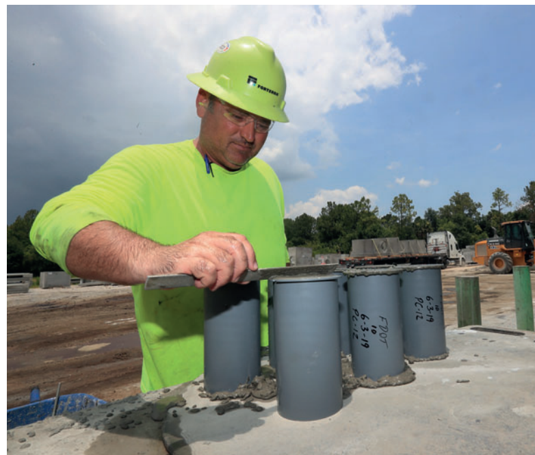
Fig 12: Superior high early strength, verified through cylinder tests, provides greater confidence when stripping forms and moving products.
