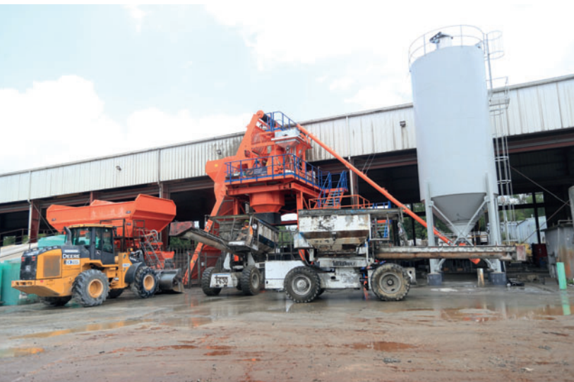
Fig 3: A Tuckerbit concrete transport vehicle pulls out with a 6 CY load from the new ACT/Wiggert concrete batch plant.
