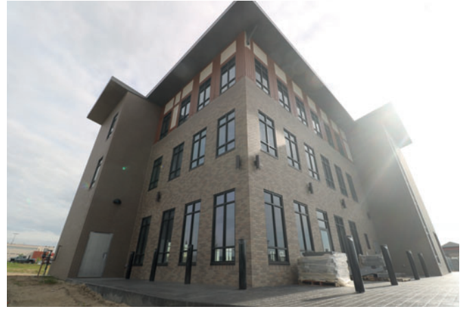
Fig. 3: The Higson Dental Clinic in Grande Prairie, Alberta, Canada, features more than 75,000 bricks cast into the insulated precast walls at the Eagle Builders production facility in Blackfalds, Alberta.
