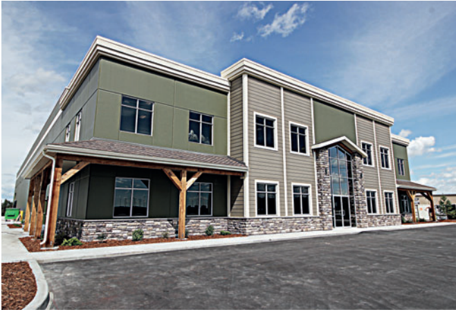
Fig. 2: Here, Eagle Builders provided a 25,500 ft 2 distribution warehouse for the Korth Group. The project included nearly 200 30-foot-high precast insulated wall panels.
