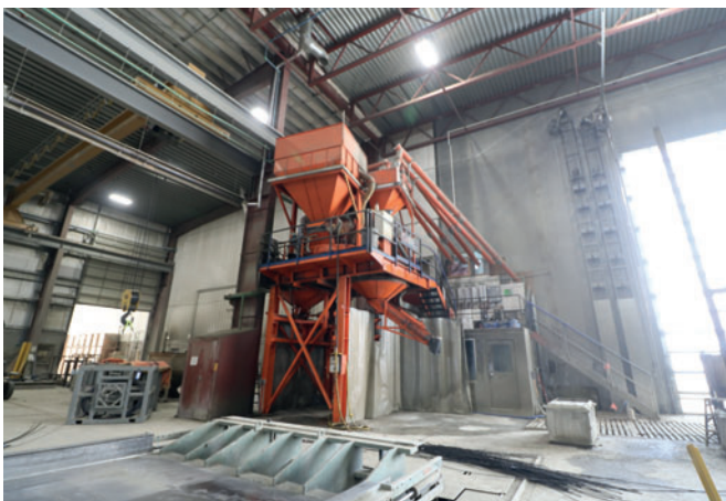
Fig. 7: Eagle Builder's 2012 expansion resulted in an increase in plant floor space from 55,000 to 100,000 ft 2 and featured the addition of an advanced computer-controlled batch plant from ACT/Wiggert that enabled the firm to convert to SCC and thereby eliminate most vibration equipment.
