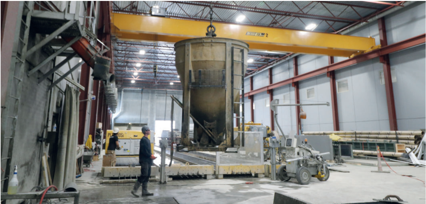
Fig. 9: Multiple overhead bridge cranes and crane buckets have been used to replace concrete carts there were required in the old plant. The new fully automated ACT/Wiggert batch plants allow the batch plant operator to focus on crane operation and timely concrete placement.
