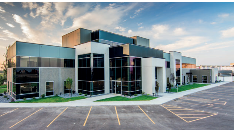
Fig. 1: Eagle Builders' new office building was completed and occupied by the firm last August. The facility features the firm's precast insulated wall panels, hollow-core slabs, and other precast components.
