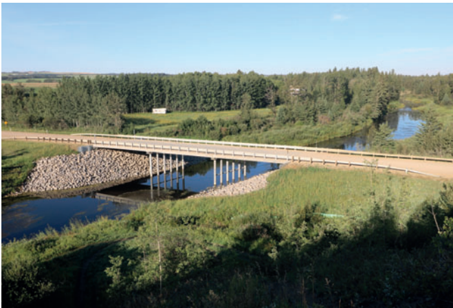
Fig. 4: Road bridge in the county of Lacombe, Alberta, Canada. Eagle Builders manufactured 24 girders for this project at its 150,000 ft 2 production facility in Blackfalds, Alberta.
