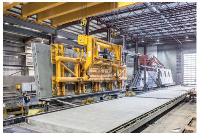
Fig 8: Insulated wall panel casting beds inside the 150,000 ft 2 Eagle Builders plant in Blackfalds, Alberta, Canada. Once panels are stripped, a vacuum-powered lift from Aerolift is used to lift the finished panel from its casting bed.
