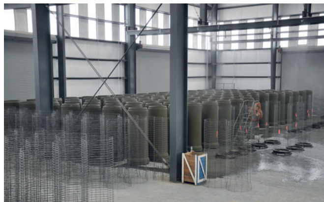
Fig. 2: A special hydraulic operated forklift attachment picks the jackets, opens and closes the seam and pallet retainers. This mold-stripping method affords tight spacing of green pipe. Here, dozens of green concrete pipes stand at attention in the curing area before being moved to the storage yard.
