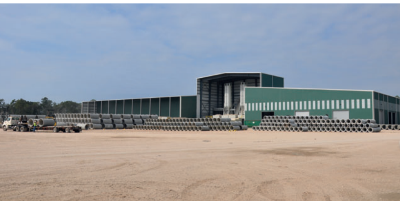
Fig. 1: AmeriTex's new plant in Conroe, Texas, USA, features state-of-art dry cast production systems and the highest level of certification available, including the prestigious QCast and TxDOT certifications.
