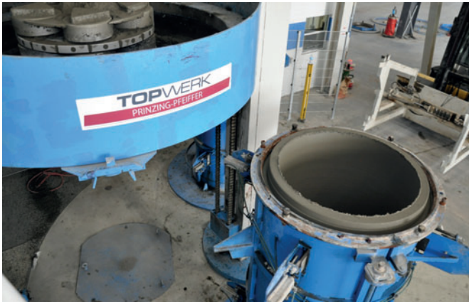
Fig. 13: Production of high quality concrete pipe is achieved by the counter-rotation pressing tool on the Radial Press, which imparts precise and tension-free reinforcing cage embedment. Here, a just-completed pipe is ready to be moved to the curing area by forklift truck.
