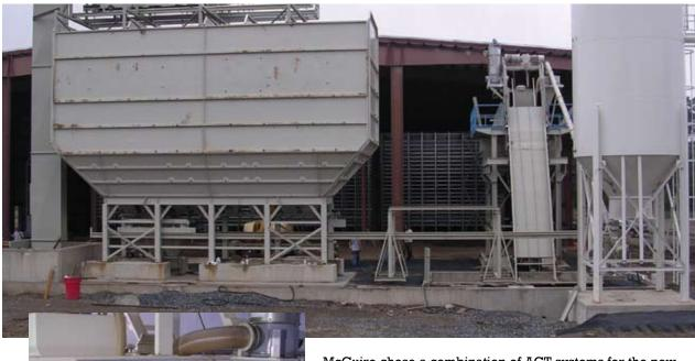
McGuire chose a combination of ACT systems for the new facility, including the Wiggert MobilMat MO80 - 5 - PCS with a high intensity planetary countercurrent mixer, and a fully automatic Würschum COM 70-3 pigment metering system.
