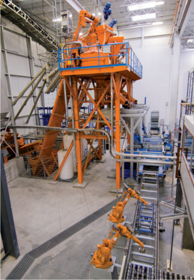
The Stonedge plant wet line is shown here, prior to plant start-up. Two Automacac Color-I color application robots stand ready in the foreground, while the ACT MobilMat Mo2250-750 concrete batching system looms over the line in the background. Continuous automatic operation is controlled by the Automacac SCADA central control.
