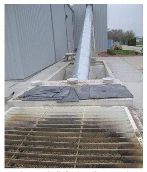
Below grade aggregate grizzly enables efficient charging of the 2-compartment indoor aggregate silo directly from a truck or frontend loader – no double handling required.
