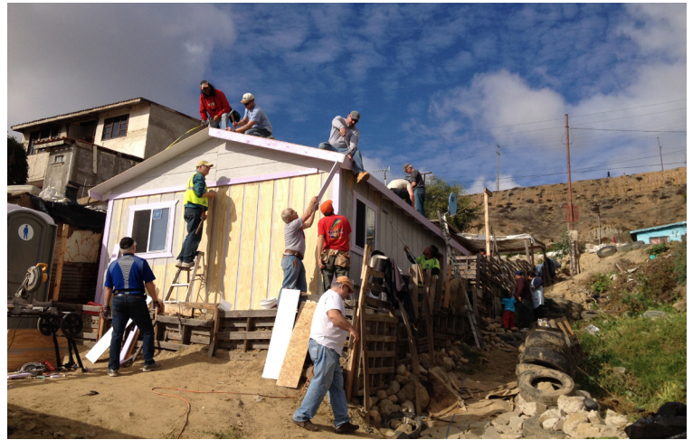
The crew painting and roofing the new house
