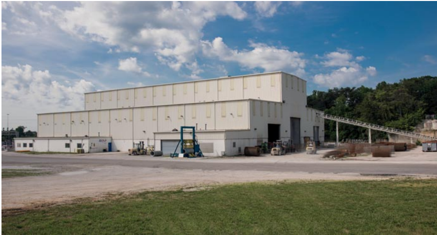
The aggregate conveyor (at right), reused from the previous batch plant, is supplied from an existing charge hopper. Aggregates are deposited into one of three compartments in a 195-ton indoor aggregate storage bin system. The 70,000 square foot Jessup, Maryland, facility produces a mix of round and horizontal elliptical precast concrete pipe, as well as box culverts and other precast products.
